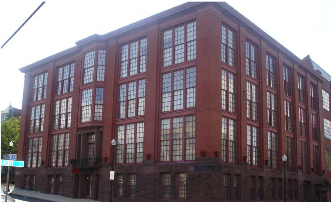
The McFarland Press Building constructed in 1906 was meticulously rehabilitated in the 1990's. Notice that the character defining windows have been repaired and replaced in-kind.
