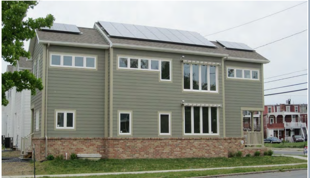
A newly constructed home in the Mount Pleasant neighborhood fitted with solar panels.
