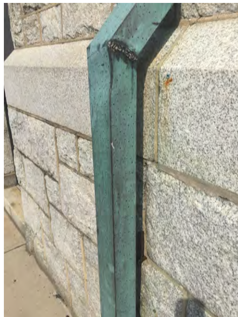
This historic copper gutter is a character defining feature and should be preserved.
