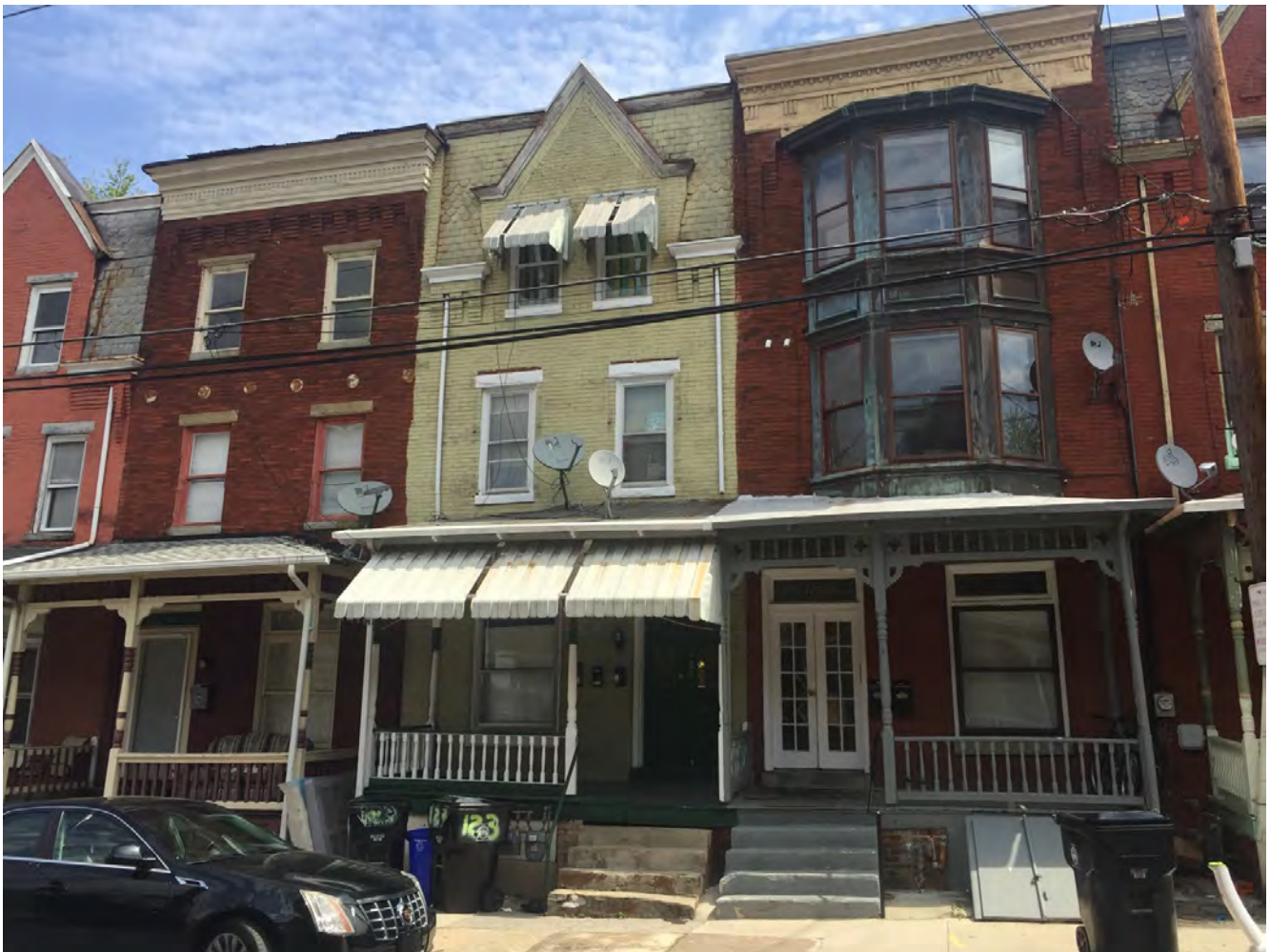
This historic streetscape is diminished by the installation of several satellite dishes. Such utilities should not be mounted on primary facades.
