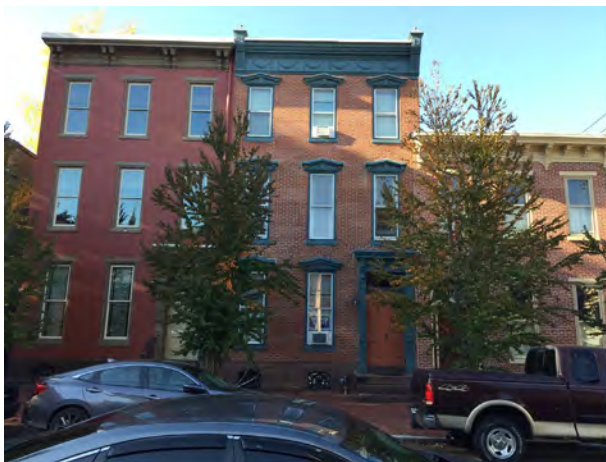
Example of Primary Facades
