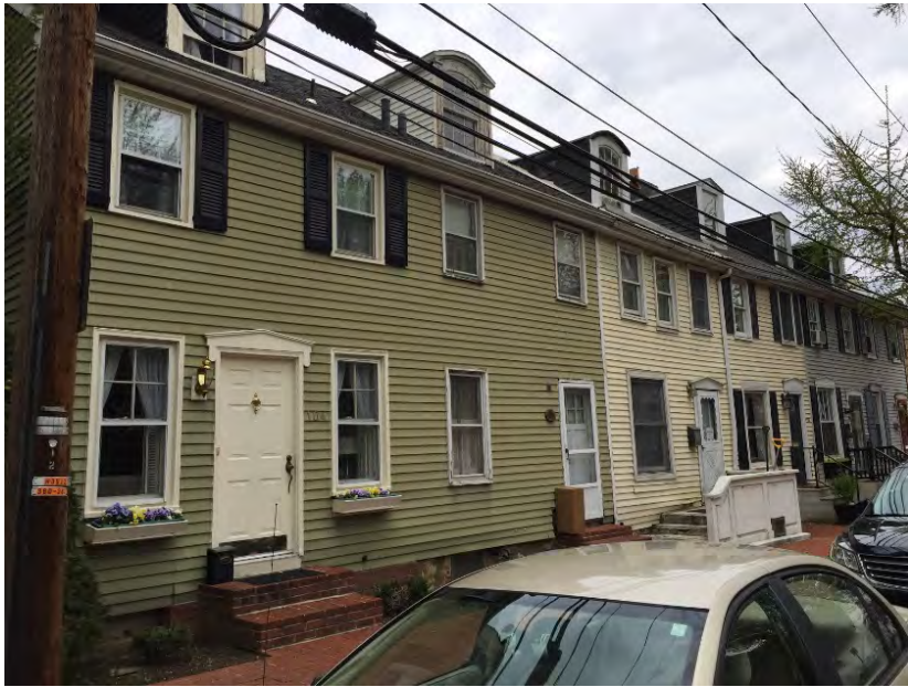
Here is a row of homes which have lost much of their historic integrity. many of these homes had vinyl and aluminum siding installed. These contemporary materials have eliminated and destroyed original historic features.
