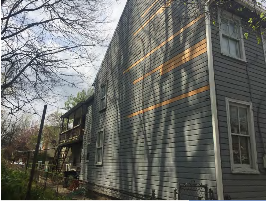
This homeowner on 2nd Street has replaced deteriorated wooden siding in-kind with new wood siding.
