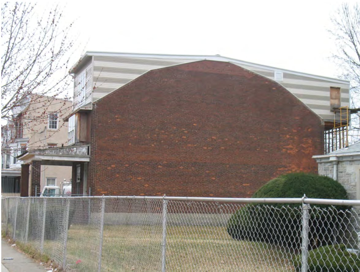
Even though not in a historic district, this large roof addition on this property on North 6th Street is wildly inappropriate as it destroys the form of the original gambrel roof. The addition removes the original features on the primary facade and destroys the historic integrity of the property. This addition is not appropriate.
