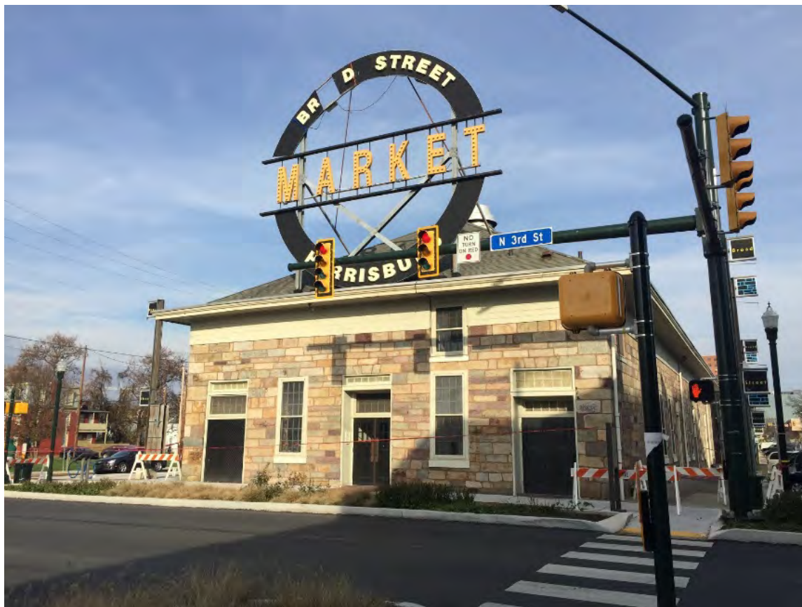
Constructed in 1863, the Broad Street Market's stone building is a prime example of how historic preservation enhances the economic development of communities.
