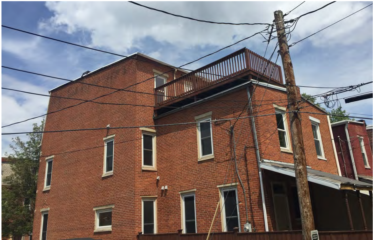
A rooftop deck was recently installed on this Uptown home. Rooftop decks can have an impact on property values. Rooftop decks have a large visual impact on the historic district and usually require HARB review.
