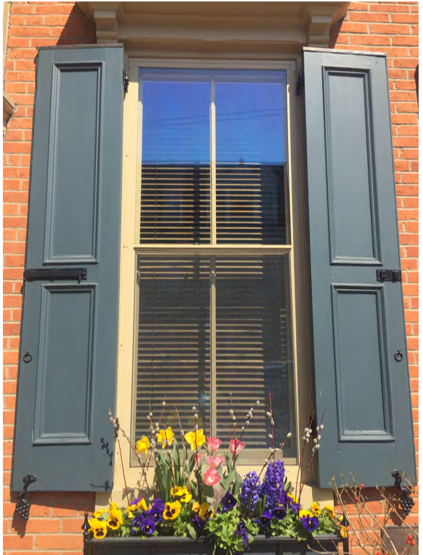
This historic window has been restored and is complemented by historic wooden shutters, hardware, and a new storm window.
