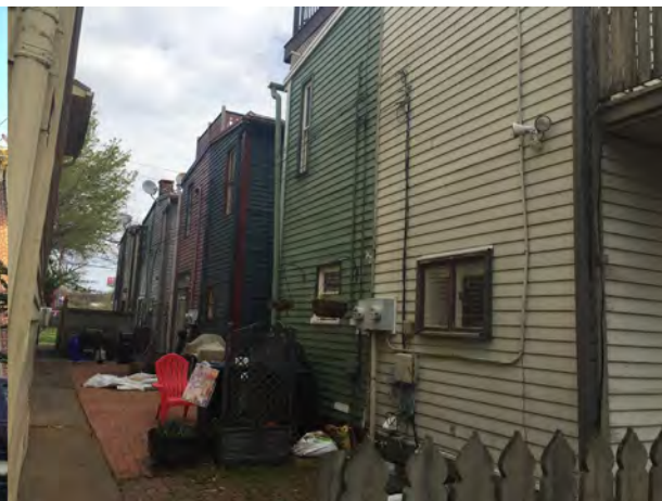
Example of Secondary Facades
