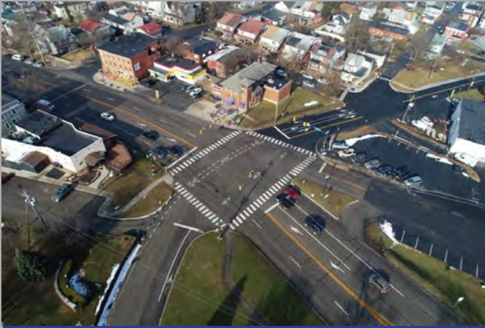
State Street at Civil War Drive has been remarked to include a bike lane and high-visibility crosswalks
