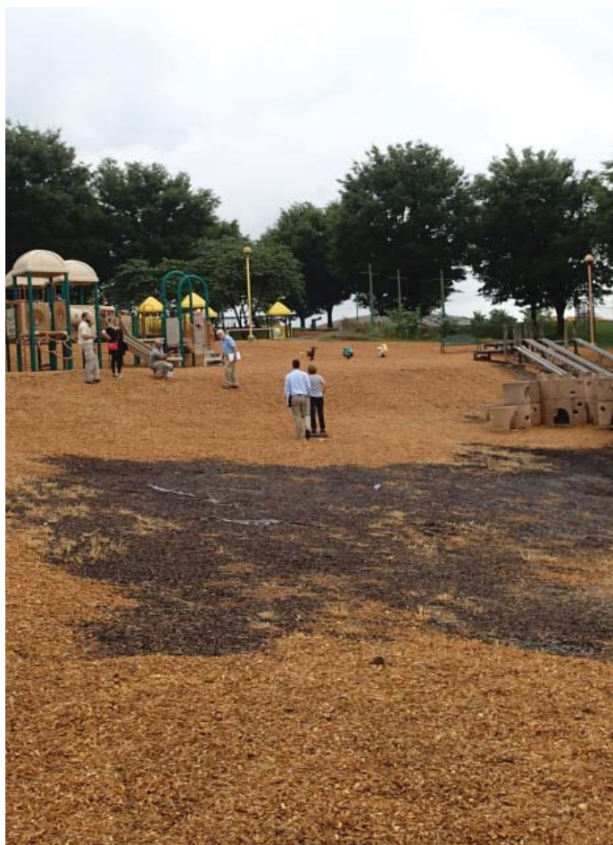
The existing playground equipment is dated and some structures exhibiting wear
